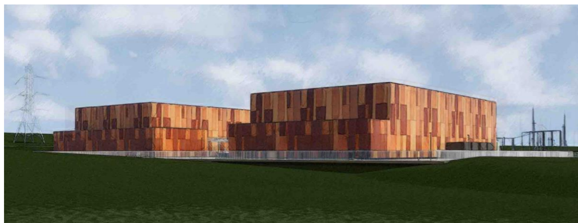
Plate 4.5 – Vertically arranged brown cladding
