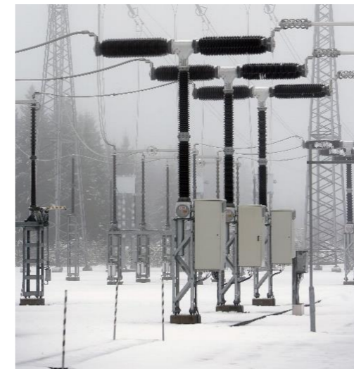
Plate 5.9 – Typical HVAC Circuit Breaker Image: ©ABB
